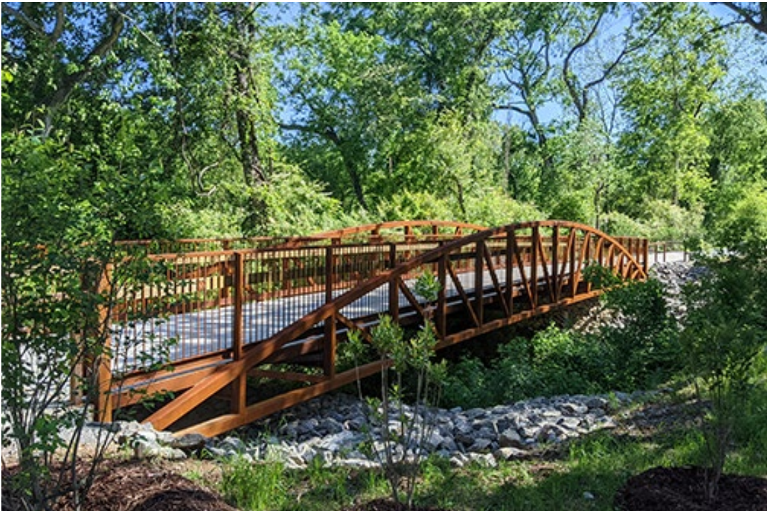
Multiuse Bridge in Etowah River Park Image Source: Destination Cherokee, 2019
