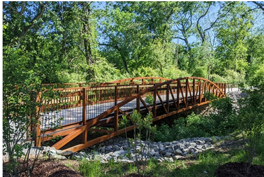
Multiuse Bridge in Etowah River Park
