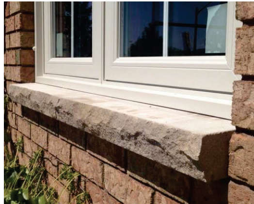
Cut stone window sill detail
