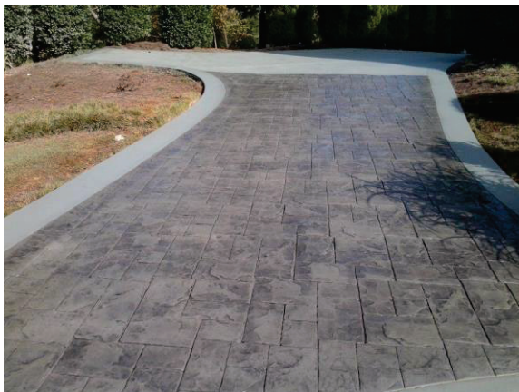
Stamped concrete with integral color – slate pattern at driveway
