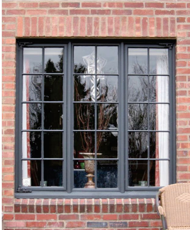
Casement window installation in brick wall with 6" recess from face of brick wall to face of window.
