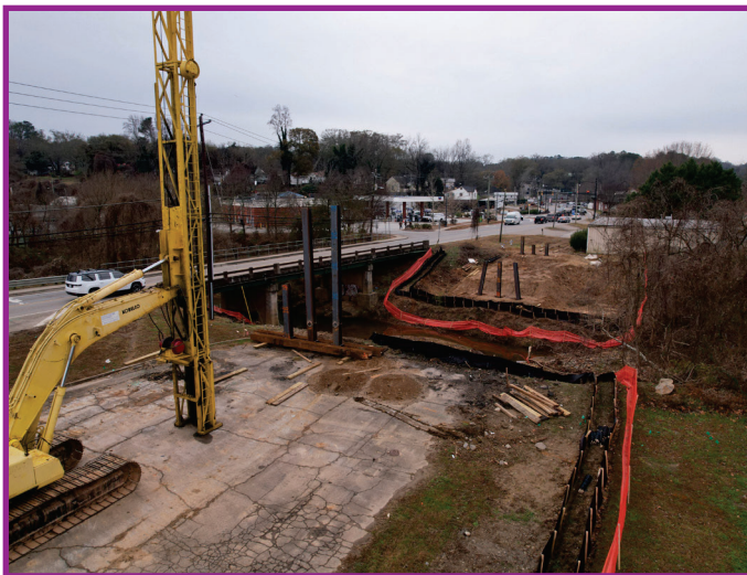
Canton Creek pedestrian bridge construction management
