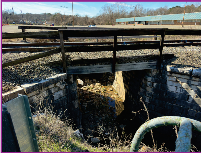
Existing masonry culvert
