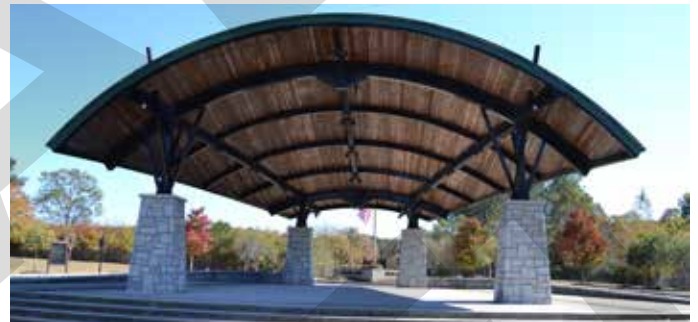
Existing stage in Etowah River Park
