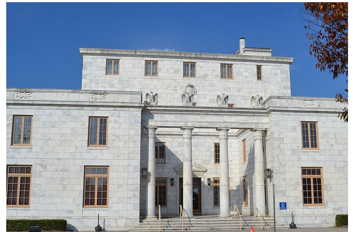
Historic Cherokee County Courthouse
