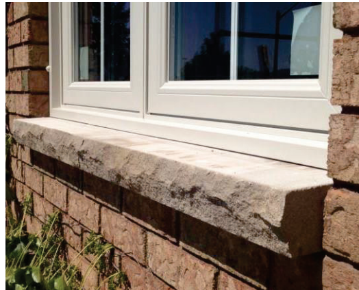
Cut stone window sill detail
