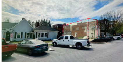
251 EAST MAIN STREET - Building Site
