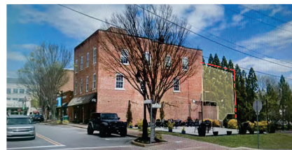
EAST MARIETTA STREET - Looking North
