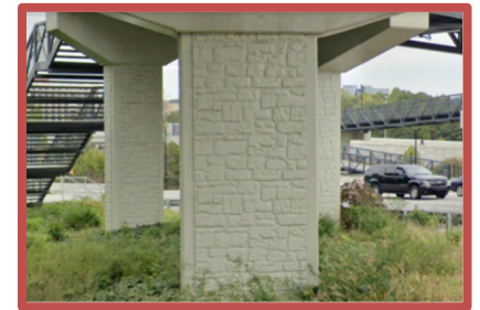
Hammerhead Bent Enhanced with Decorative Formliner.
