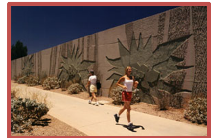
Retaining Wall Enhanced with Color and Custom Formliner.
