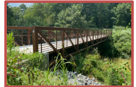
Weathering Steel Prefab Truss.
