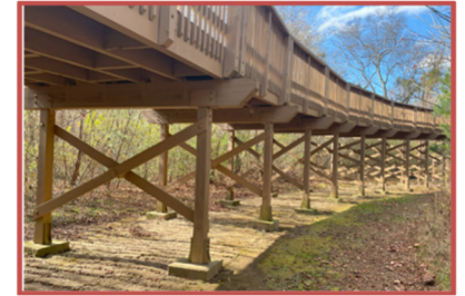
Elevated Timber Approach
