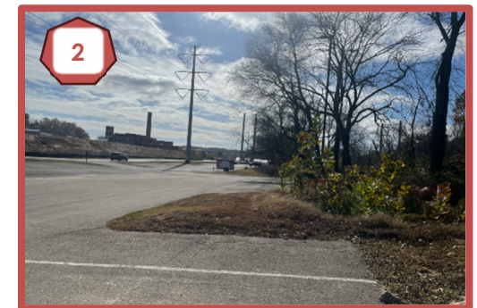
Image Showing The Mill on Etowah, the Overhead Transmission Line, Looking South from the East Bank of the Etowah River.
