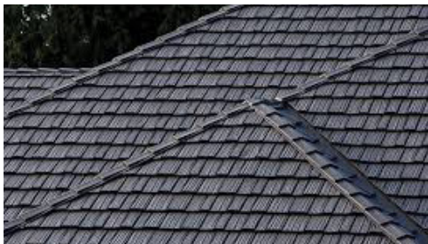
Stamped metal shingles are an appropriate, long-lasting, and quality material for late 19 th and early 20 th century houses.
