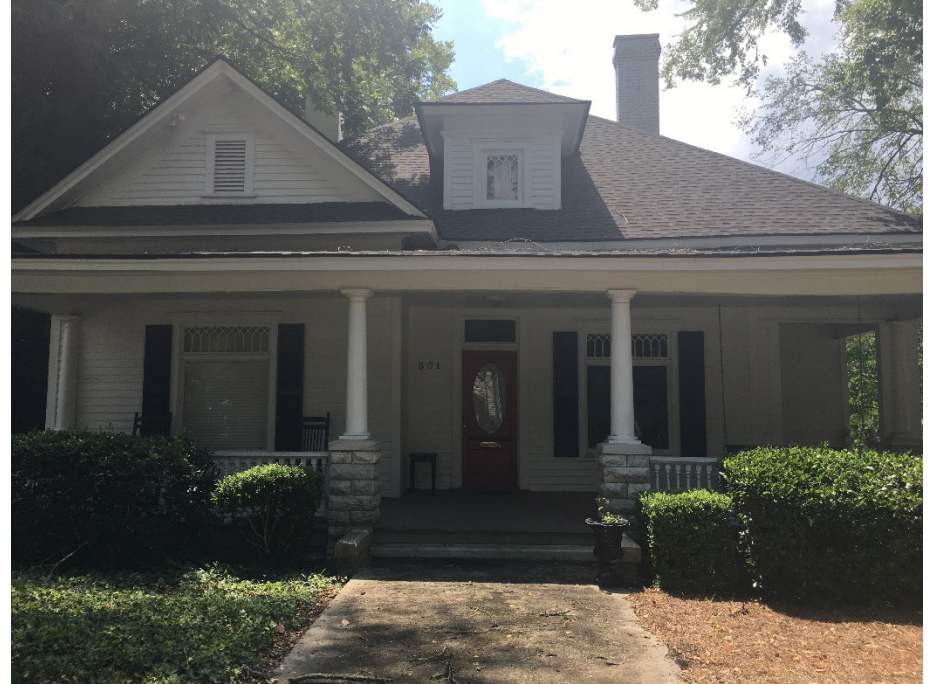
501 East Main Street is a local example with elements of the Queen Anne style.
