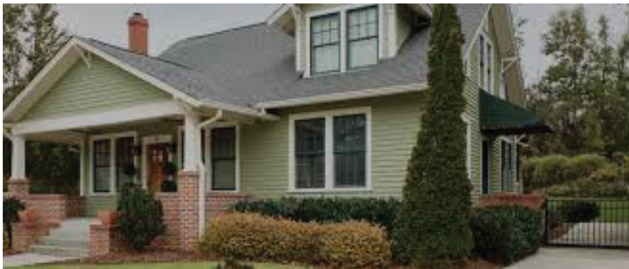
Windows in groupings or having a rhythm of repetition are significant character defining features to the form and style of a home.
