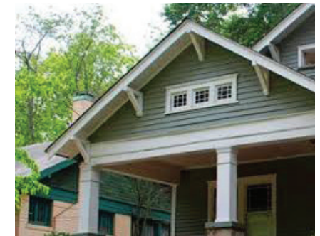
Brackets, eave overhang, and verge board (shown on the front gable end of a Craftsman-style bungalow) all help define the style and denote construction technology of the time a home was built.
