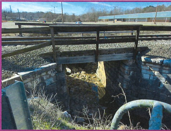
Existing masonry culvert
