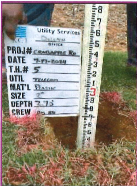
Example Test Hole by KCI
