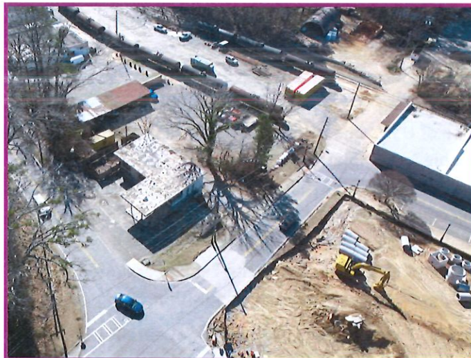
Marietta Road at W Marietta Street and Railroad Street
