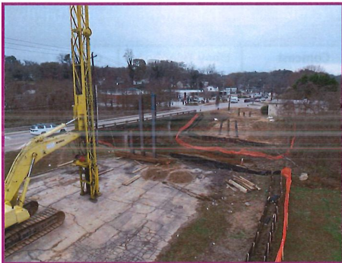
Canton Creek pedestrian bridge construction management
