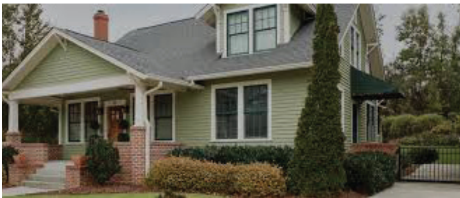
Windows in groupings or having a rhythm of repetition are significant character defining features to the form and style of a home.
