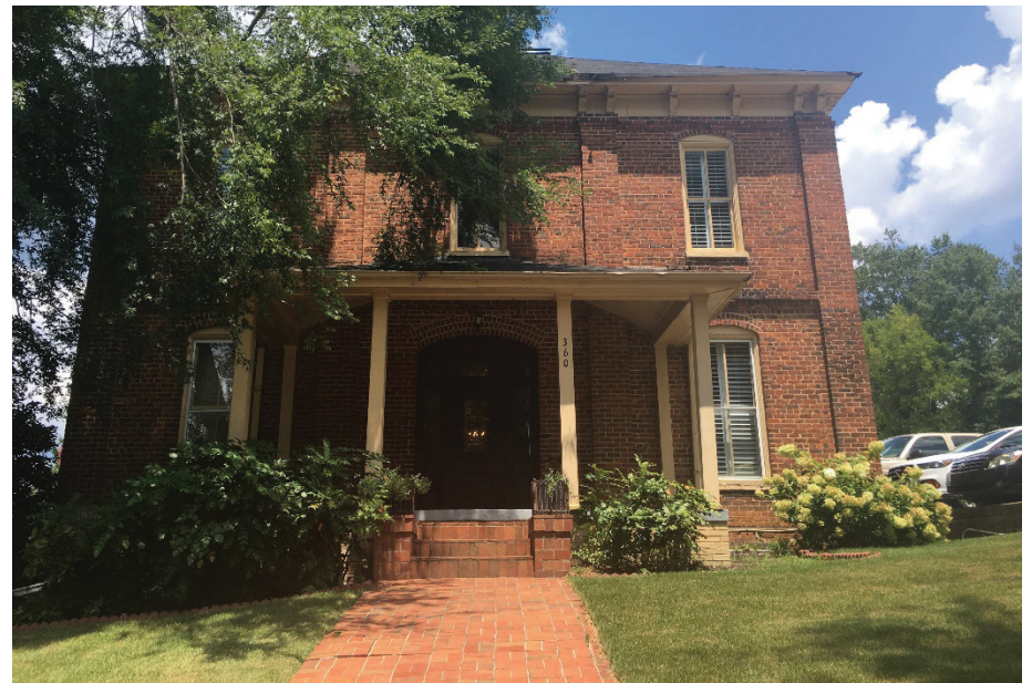
360 West Main Street is a local example with elements of the Italianate style.
