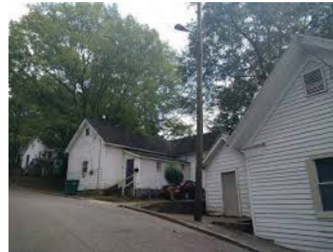
The Cotton Mill Village in downtown Canton (middle and bottom). The Mill Village was built around 1900 and provided housing for the workers of Mill #1. The Mill Village homes are located along Riverdale Circle, Middle Street, Hill Street Circle, Hill Street, Academy Street, and Railroad Street.
