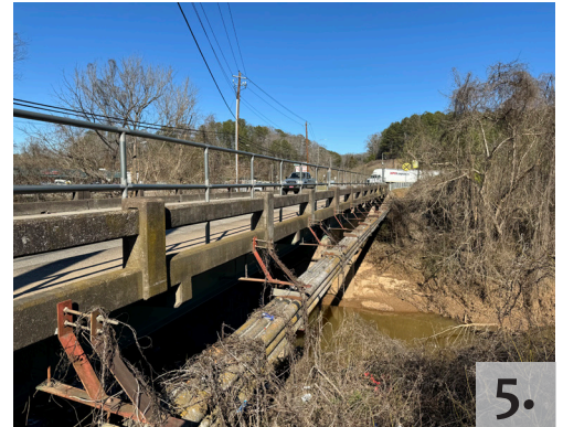
5: Telephone conduits attached to bridge 6: Gas line attached to bridge
