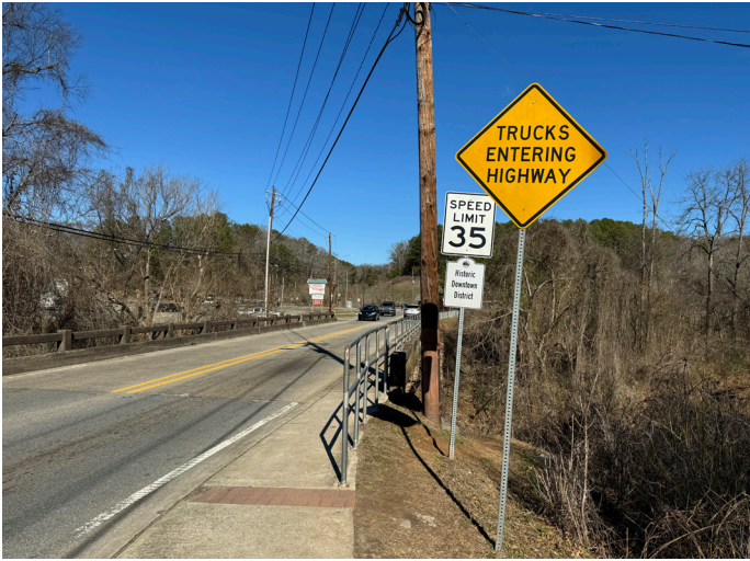
Existing sidewalk- east side of bridge
