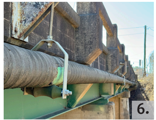
5: Telephone conduits attached to bridge 6: Gas line attached to bridge
