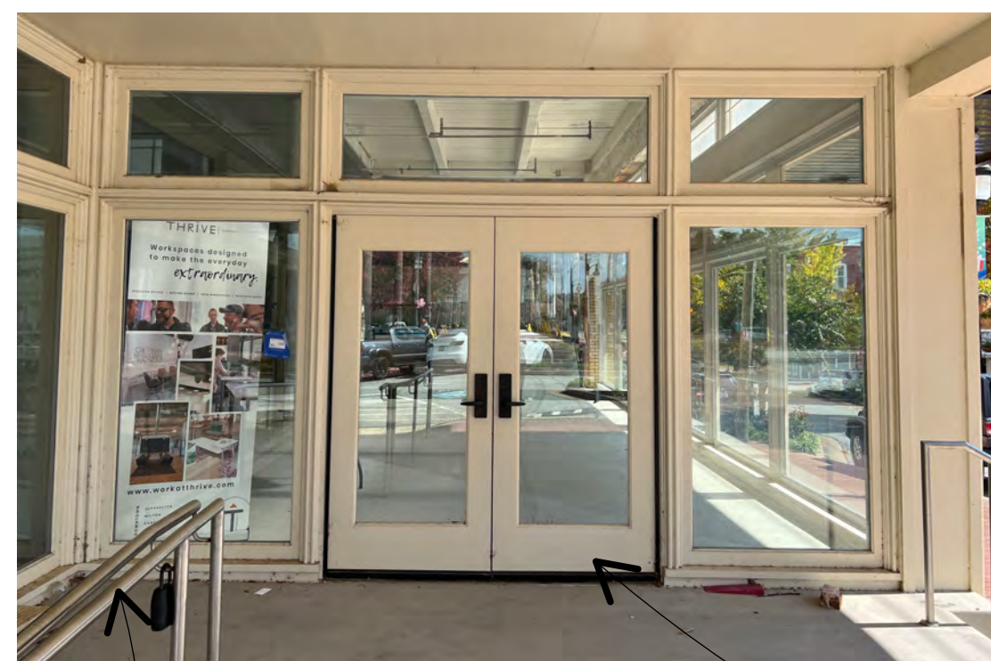
7 EXISTING STOREFRONT IMAGE
