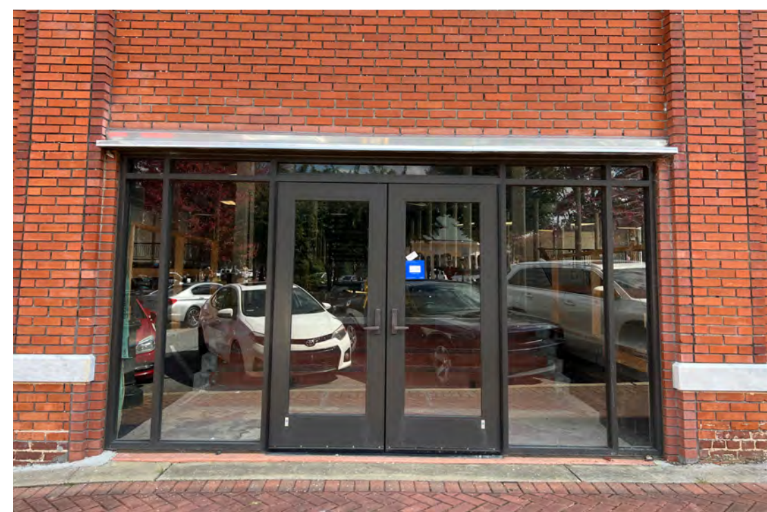
8 EXISTING STOREFRONT IMAGE - LOCATION "A"
