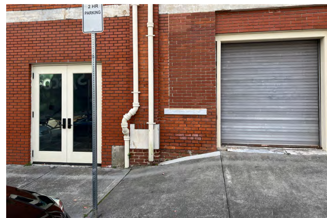
9 EXISTING EXIT DOOR IMAGE - LOCATION "B"
